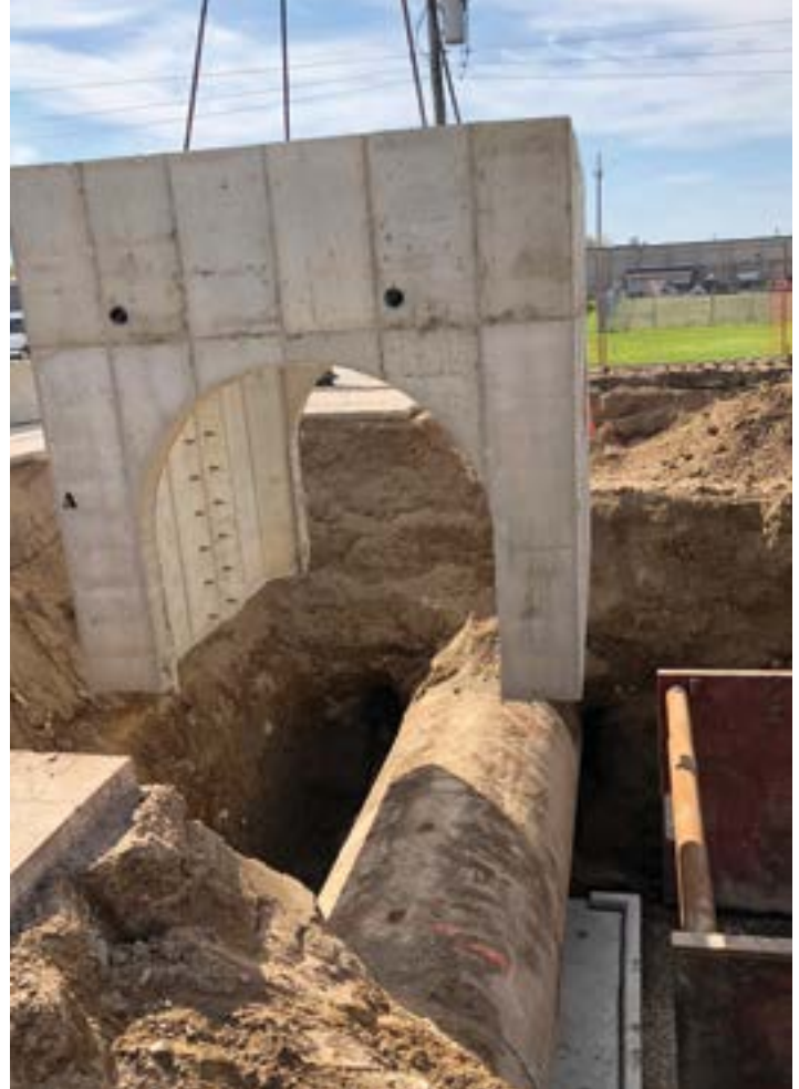
Custom doghouse structure being lifted into place.
